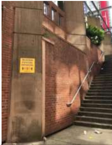
Signage for pedestrian coming from Betty Lane
